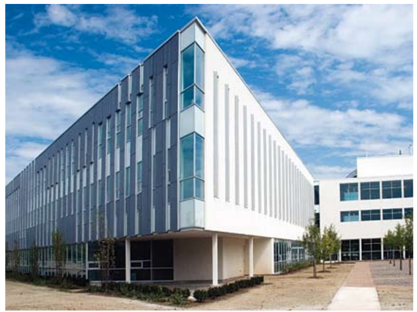
The Regional Municipality of Niagara recently expanded its Campbell East, Niagara Region headquarters in Thorold, Ontario and incorporated such energy efficient features as high thermal resistance in the walls and roof, high performance windows, efficient condensing boilers, occupancy sensors for lighting efficiency, and low flow water fixtures, among others. (Photo: Enermodal Engineering Ltd.) Photo courtesy of the Canada Green Building Council www.cagbc.org
