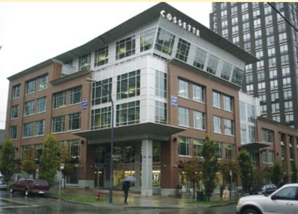
Same property: After recent redevelopment
